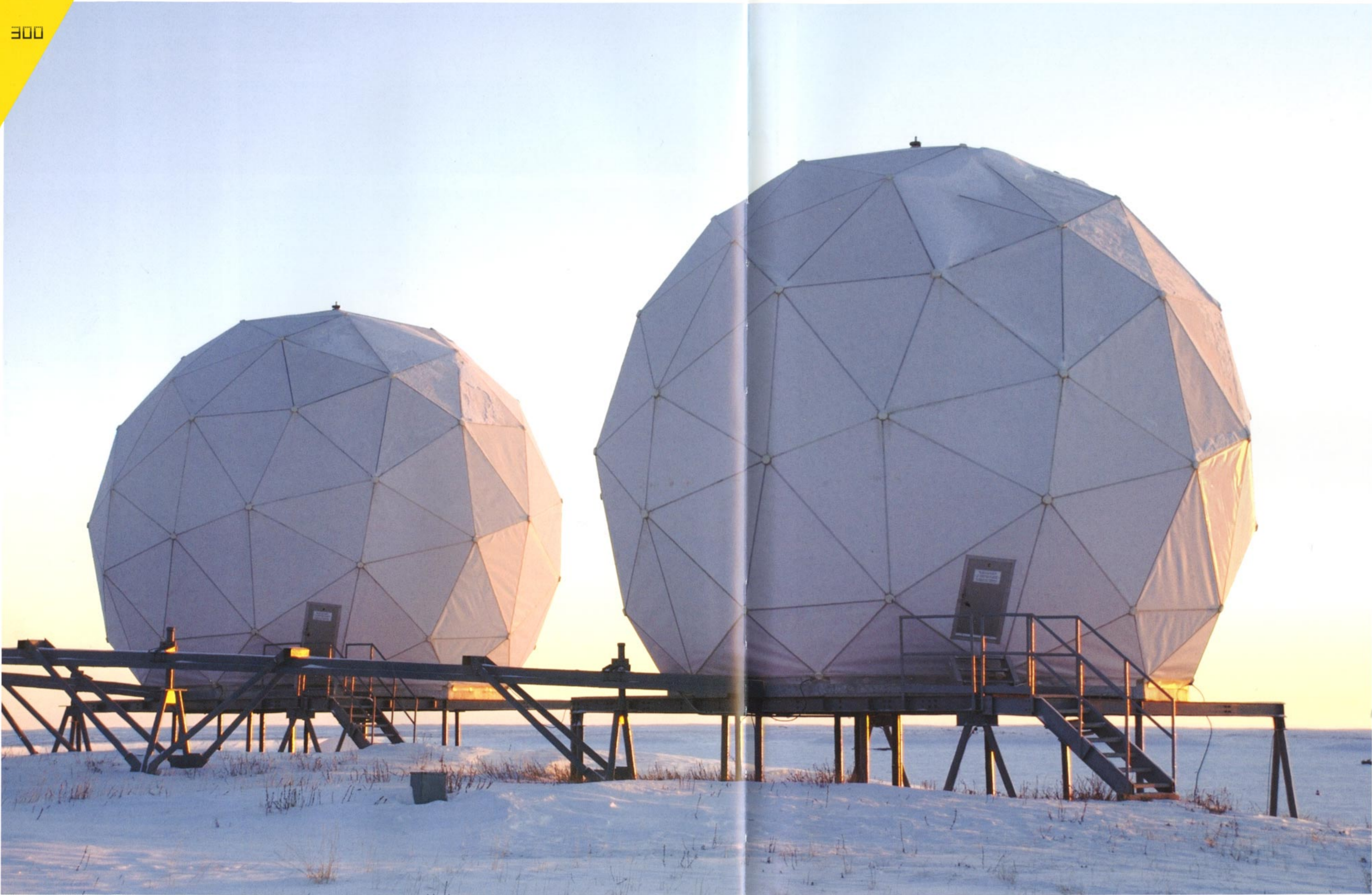
North Warning System Radomes, historic site of BAR-3 DEW Line, Tuktoyaktuk, Northwest Territories, Canada, 2009
